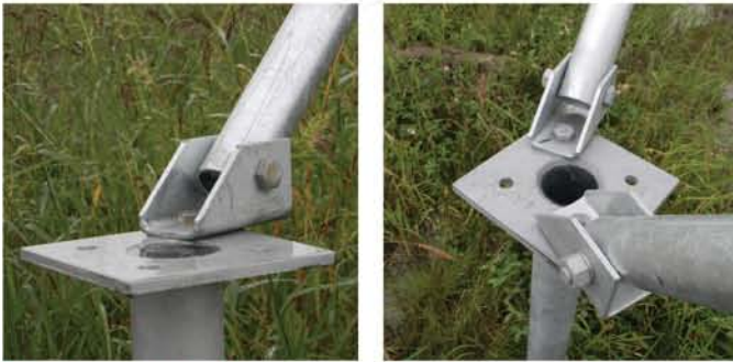
Single and double support strut connected to solar foundation pile plate.
