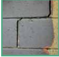
Cracks in the foundation
