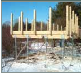
Braced brackets and placed tension anchors for support
