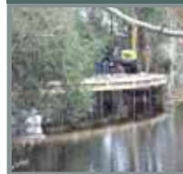
Concrete pile caps cast to support timber columns
