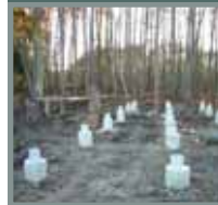
Concrete pile caps cast to support timber columns
